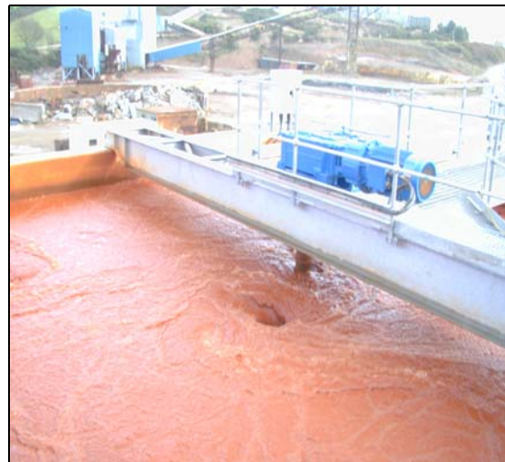
Figure 5. Stage II reactor mixer bridge
