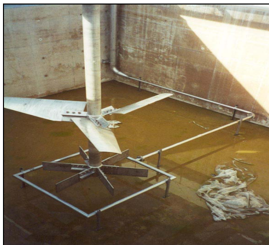
Figure 6. Stage II reaction vessel mixer
